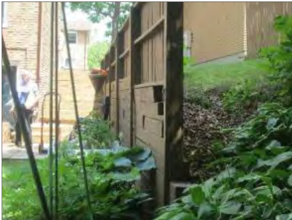
View of the wood framed retaining wall between blocks 7 and 8 which was noted to be leaning and will require replacement in the short term.
